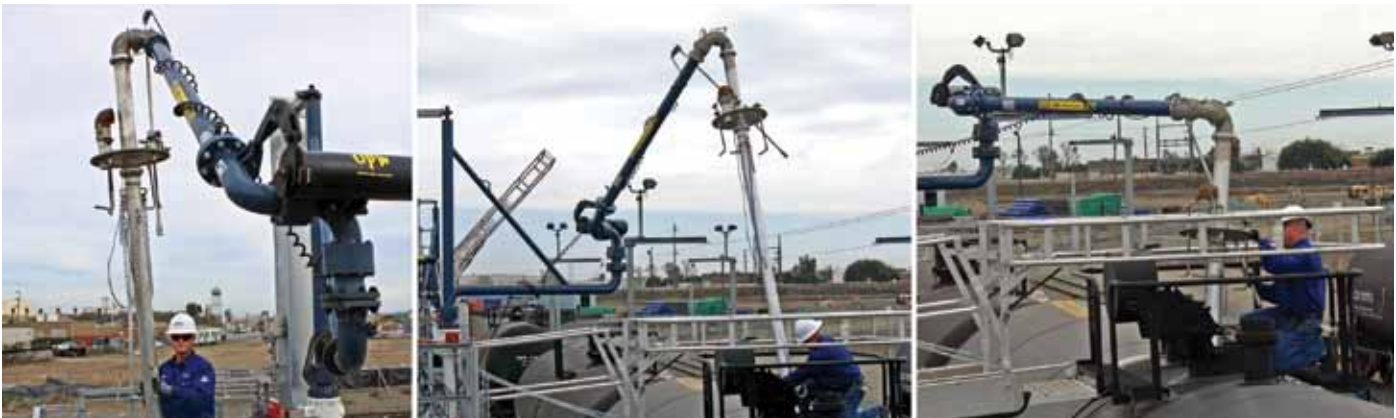
The operators of the Stockton facility required a loading-arm system with a 15-foot reach, drop tubes long enough to reach the interior bottom of any railcar and a torsion-spring counterbalance.
