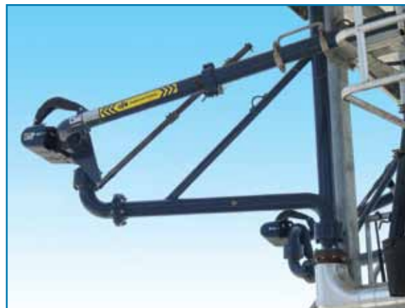
888L Loading Arm Lockdown Assembly
