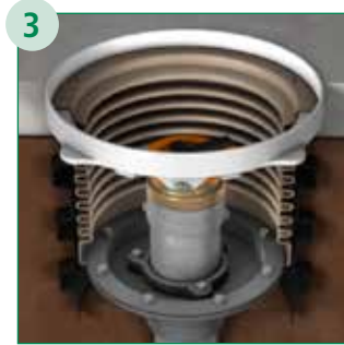
Replace Bellows, Reinstall Upper and Lower Rings
